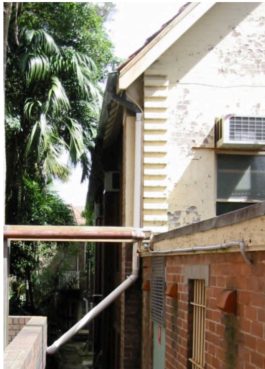
Figure 8.5.20 View to the southwest corner of the waiting room showing brick toothing suggesting that an extension was planned
